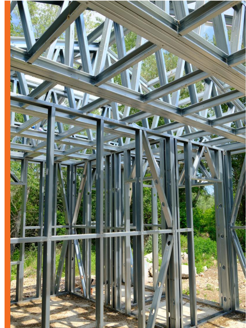
Assembled and installed LGSF panels
